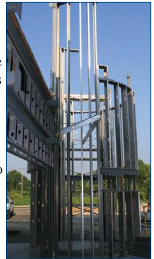
New stair tower frame at BCTC Winchester-Clark County Campus
